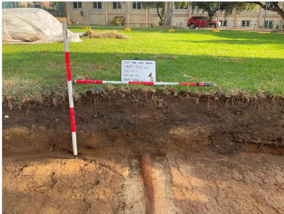
Figure 5-8: Final section showing the exposed iron service pipe [C1010].
